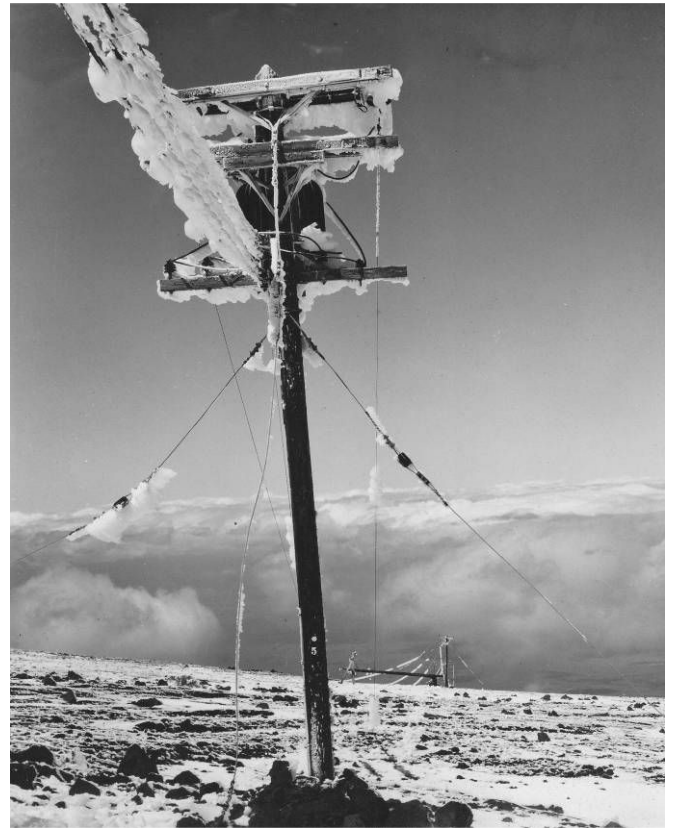
Results of an ice storm that shut down the transmitter atop Haleakalā for nearly two weeks in 1962
